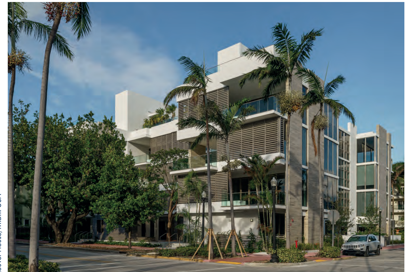
Louver House, Miami USA
